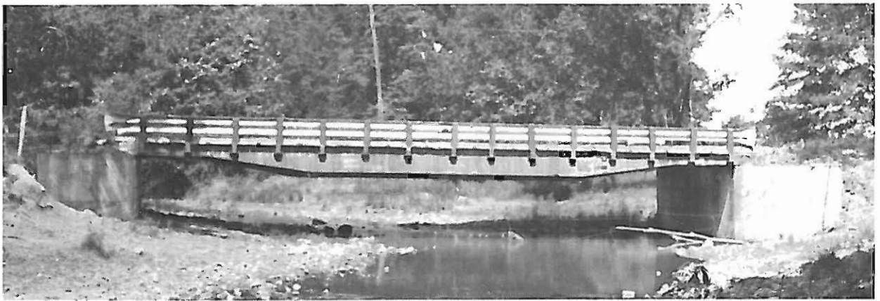
Bridge Creek Bridge on Faulkner County Road 52 north of State Highway 89.
