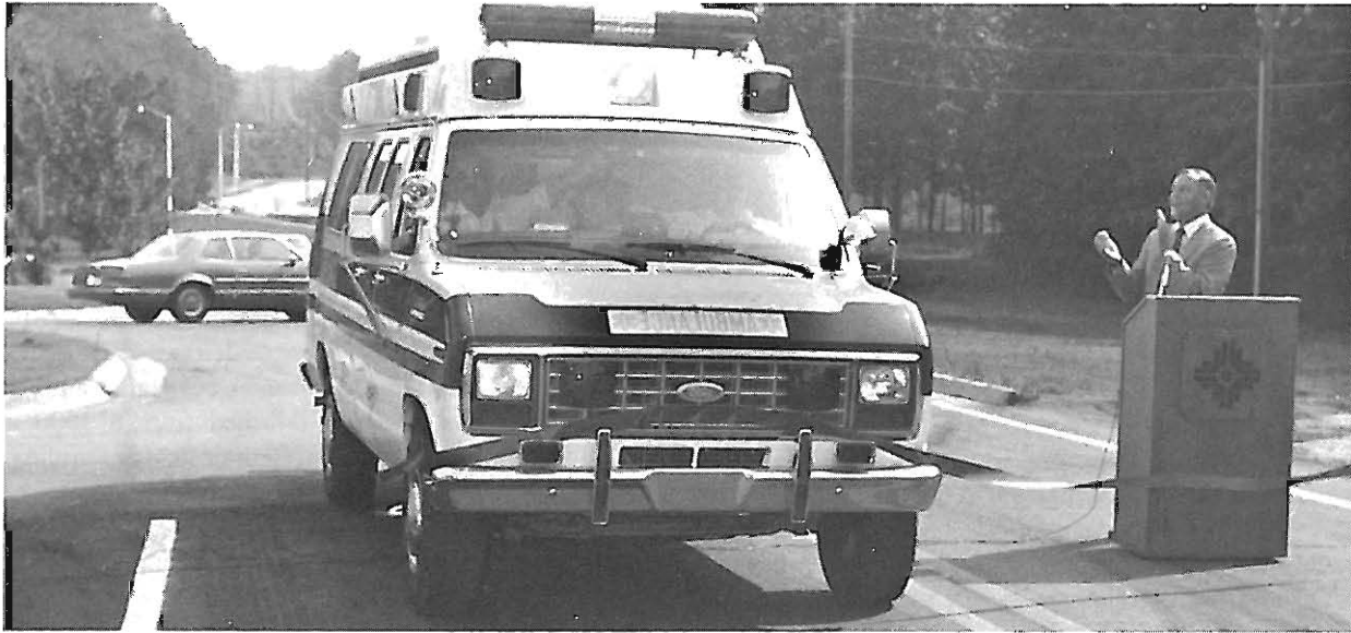
Hospital Administrator Dan Gathright applauds as an ambulance drives through the ribbon to officially open the new road.
