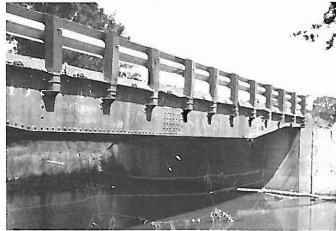
A closer look at Bridge Creek Bridge on Faulkner County Road 52.
