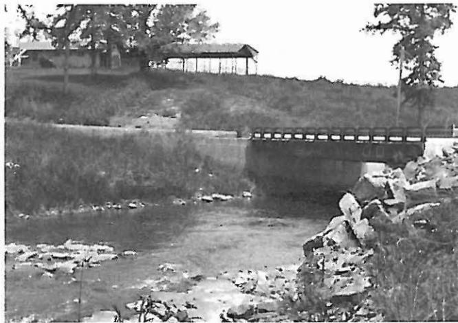
Mortar Creek Bridge on Faulkner County Road 71
